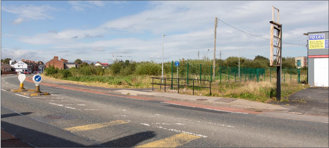
Photo 1: The site frontage to Hill Street, showing the unkempt grassland and scrub
