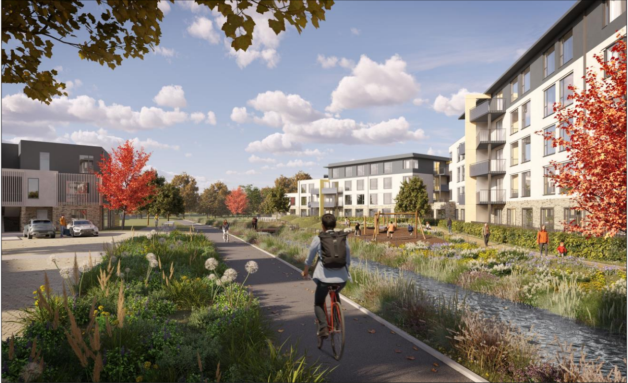
Figure 9: CGI showing the kinked alignment of Blocks B and C to the right, forming an open space alongside the Blackwater River and the greenway, and the end of a duplex terrace to the left
